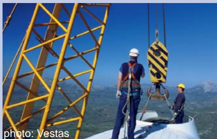
Vestas wind turbine mounting
